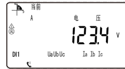
Voltage on A phase is 123.4V
