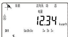
Current forward reactive energy 12.34kWh
